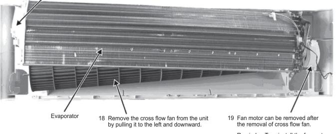
Reminder: To reinstall the fan motor, please adjust the connector to 45° with fan motor before fixing control board.
