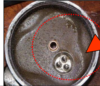
5 Upper shell water bubble mark and rusty
